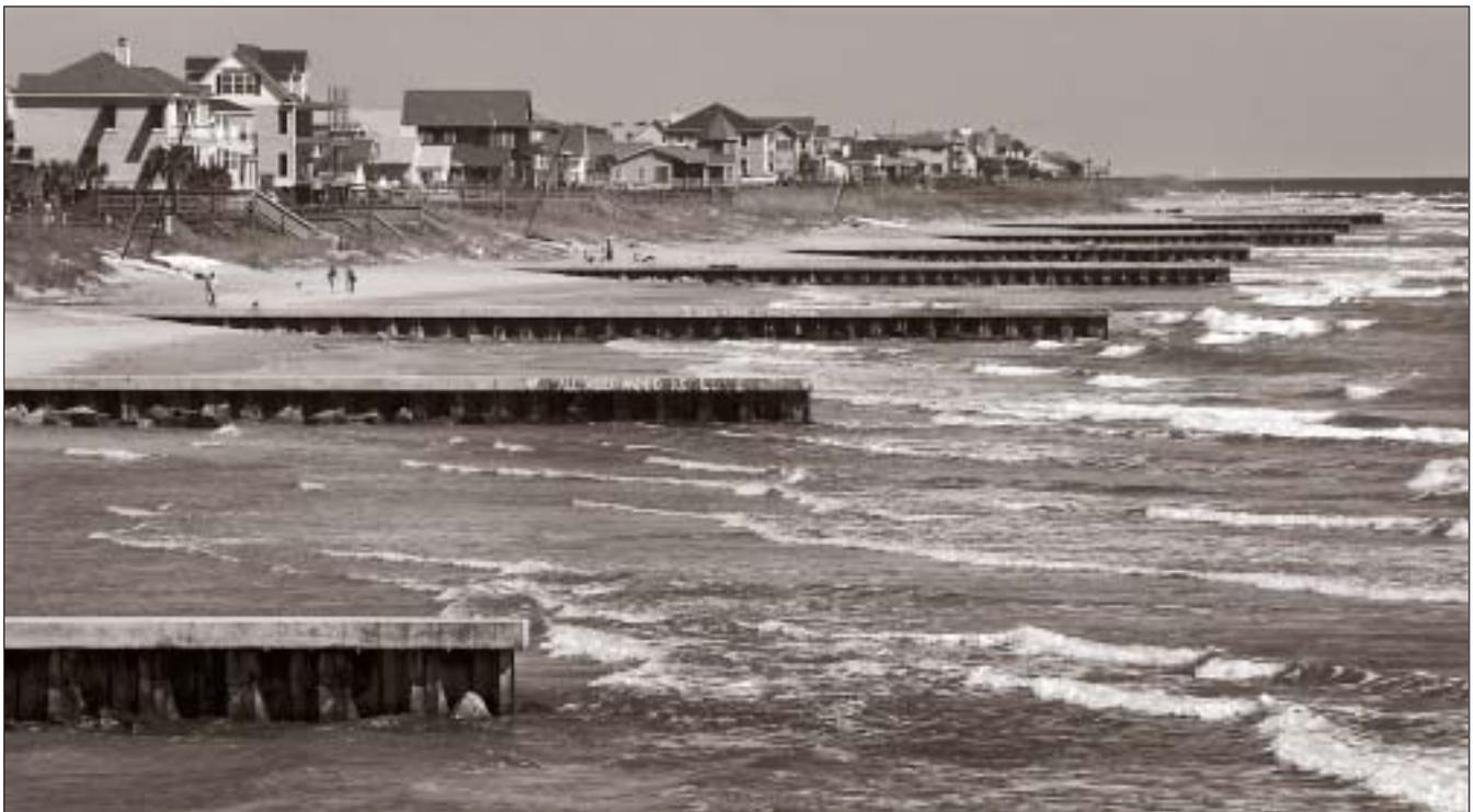
**SAND TRAPS.** Decades ago, groins—hard structures perpendicular to the shoreline—like these at Folly Beach were built in an effort to control erosion. Later, groins fell out of favor because they can starve sand from downdrift beaches. Now, under South Carolina regulations based on a recent state law, new groins can be constructed and existing groins can be reconstructed only in concert with an ongoing nourishment effort that meets special criteria. PHOTO/WADE SPEES
